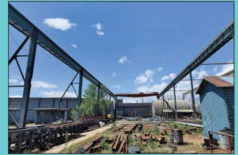
360' Approx. Crane Rail and Raceway
