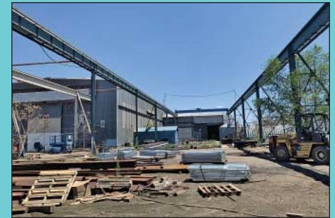
2nd View 360' Approx. Crane Rail and Raceway
