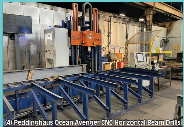
(4) Peddinghaus Ocean Avenger CNC Horizontal Beam Drills
