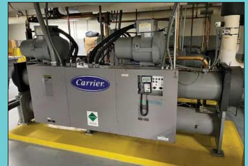
(4) 114 Ton Trane Model 30HXA116RY-640 High-Efficiency Indoor Liquid Screw Chillers
