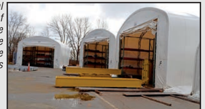
Partial View of Portable Outside Storage Sheds
