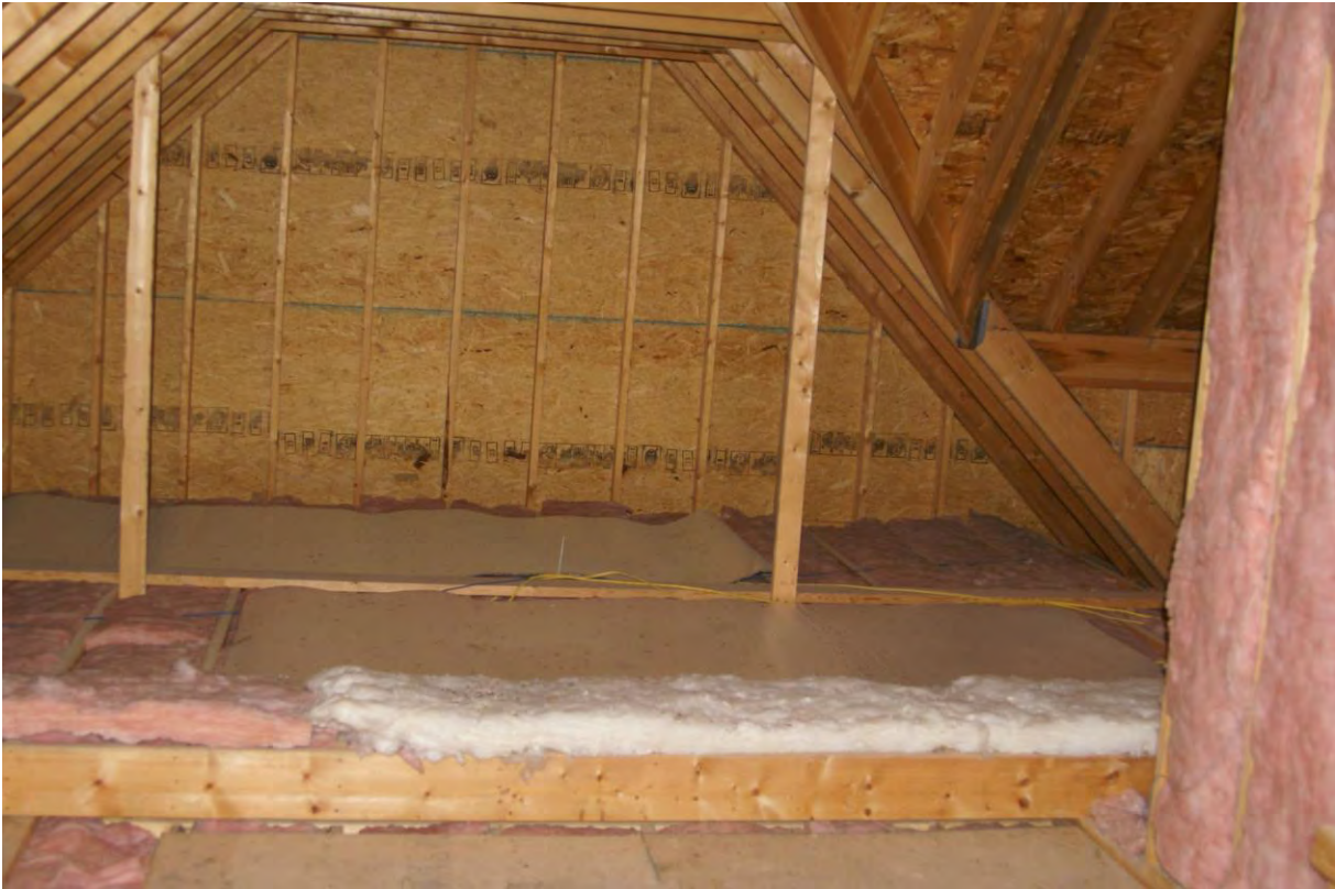
Second Floor Unfinished Space
