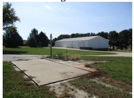
Scale w/Bldg 1 in background
