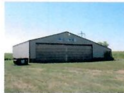
50x60 Maintenance Bldg.
