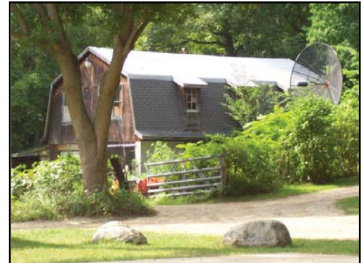
Work shop and storage building
