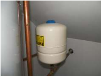
Interior Supply Piping Material: The interior supply piping in the structure is predominantly copper at the water heater and PEX plastic piping at the fixtures.
