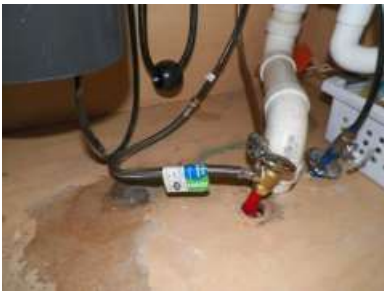
Interior Supply Piping Material: The interior supply piping in the structure is predominantly copper at the water heater and PEX plastic piping at the fixtures.
